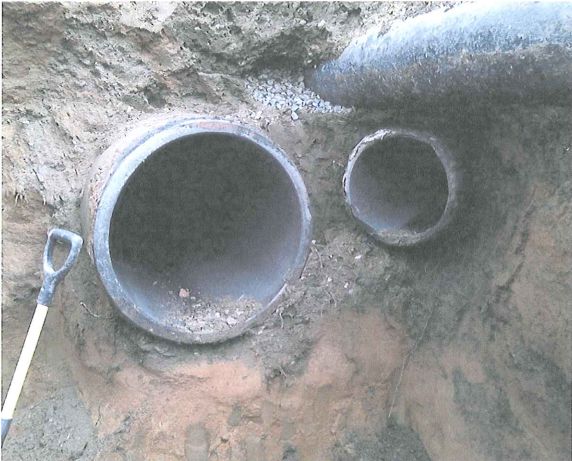
View of the Existing Storm Sewer Pipes Beneath Kings Highway East
