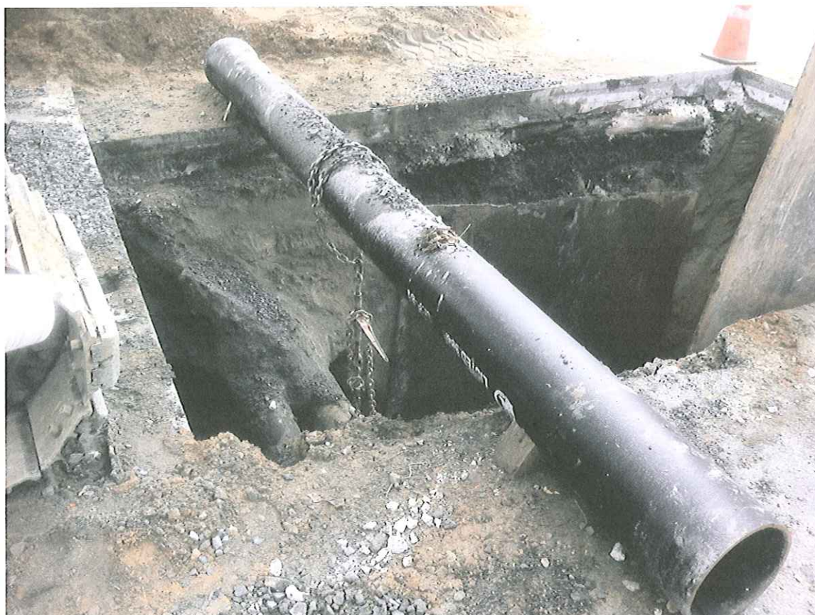
View of Temporary Support for Existing Underground Utilities Encountered During the Project
